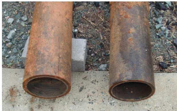
Exterior View of Force Main Pipe Installed in 1995
