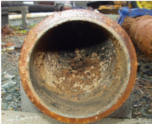
Interior View of Force Main Pipe Installed in 1995
